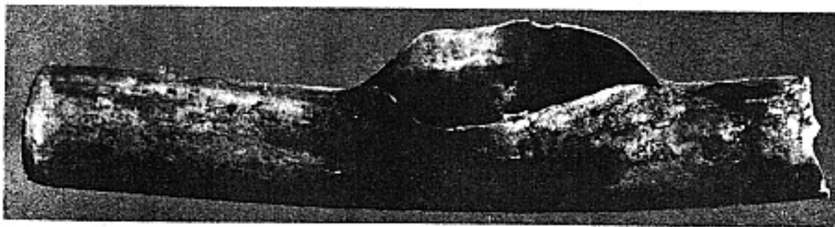
FIGURE 4-2. BOILER TUBE FAILURE CAUSED BY SCALE
