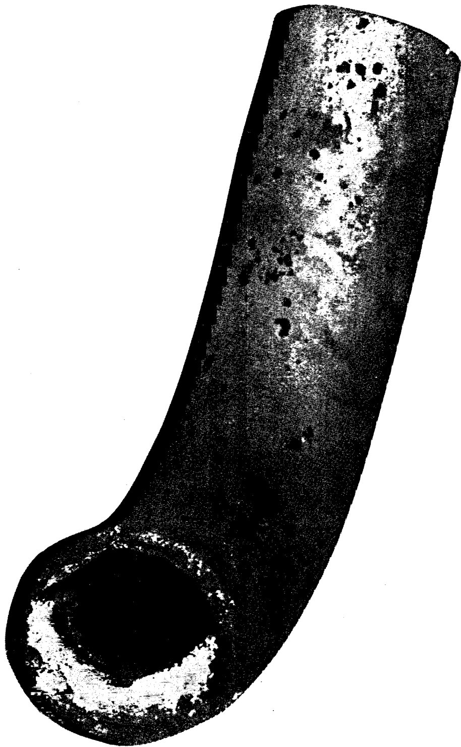
FIGURE 4-3. SUPERHEATER TUBE SHOWING CARRYOVER DEPOSITS
